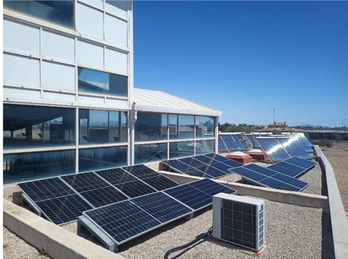
Figure 5. View of the photovoltaic panels mounted at the swimming pool roof.
