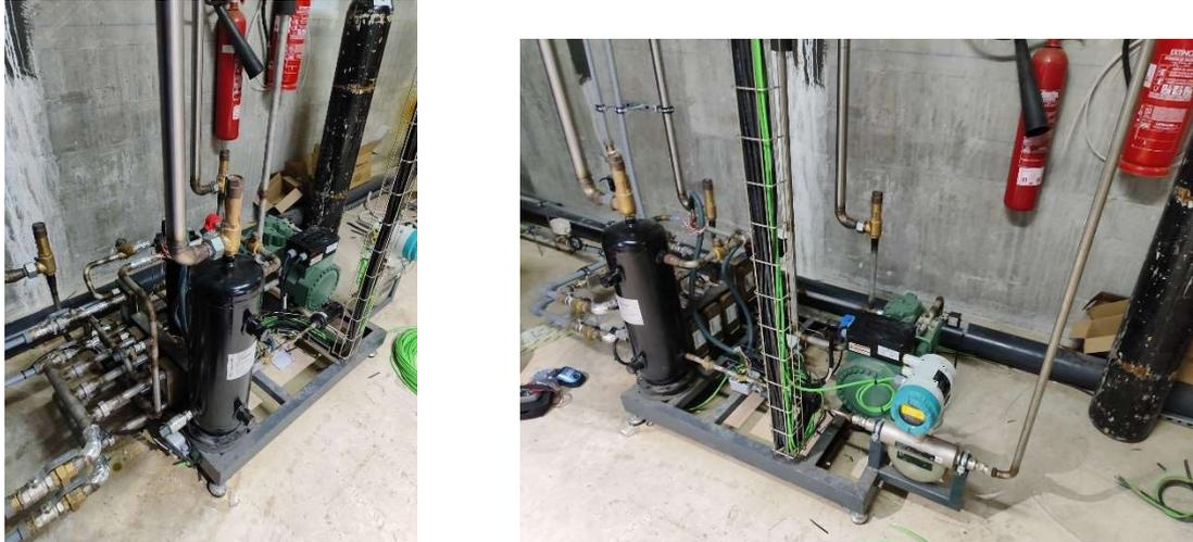
Figure 4. Two views of the heat pump constructed in the swimming pool.
