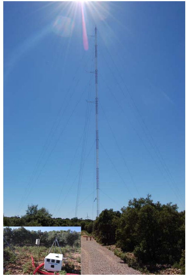
(a) Equipment at test site: WindCube (left) and Met Mast (right)
